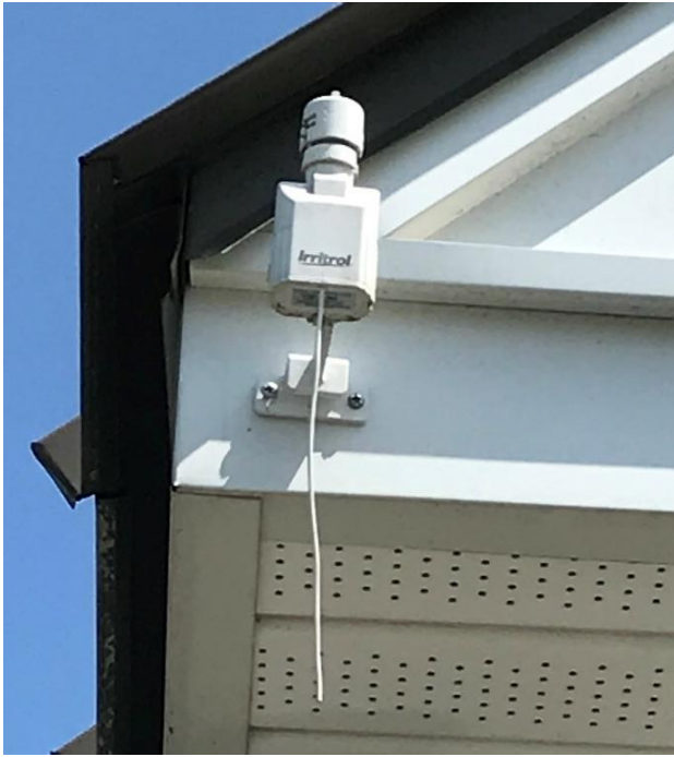
Typical wireless rain sensor located near each controller. Suspends watering during rain events.
