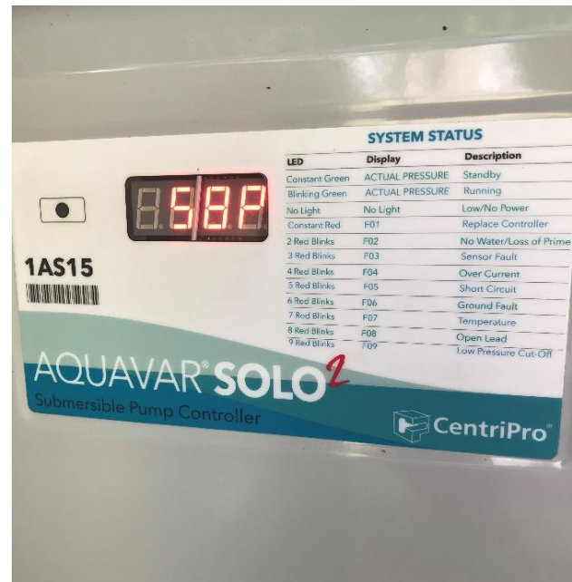
Aquavar controller - varies Pond 1 well pump speed to maintain Sloan Clubhouse irrigation system pressure
