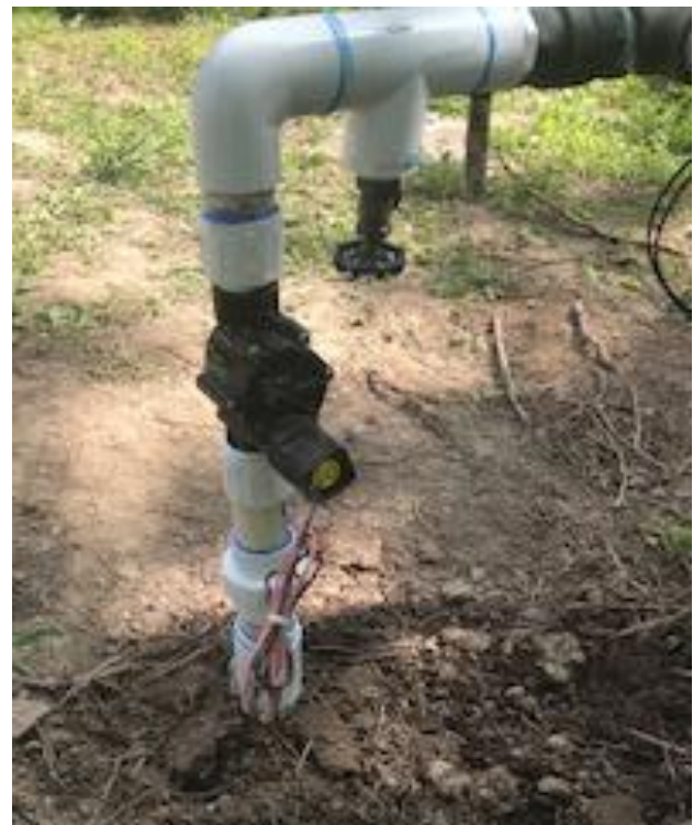
Rain Bird DC latching solenoid valve allows Pond 1 well water to pressurize Sloan irrigation system
