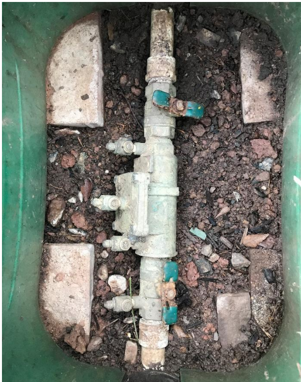
Typical subsurface valve enclosure with shutoff valves (blue handles) & backflow preventer (center)
