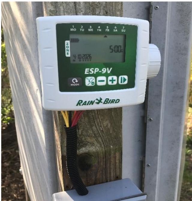
Programmable digital controller located at Pond 1 well site controls irrigation water for Sloan clubhouse as well as pond water level
