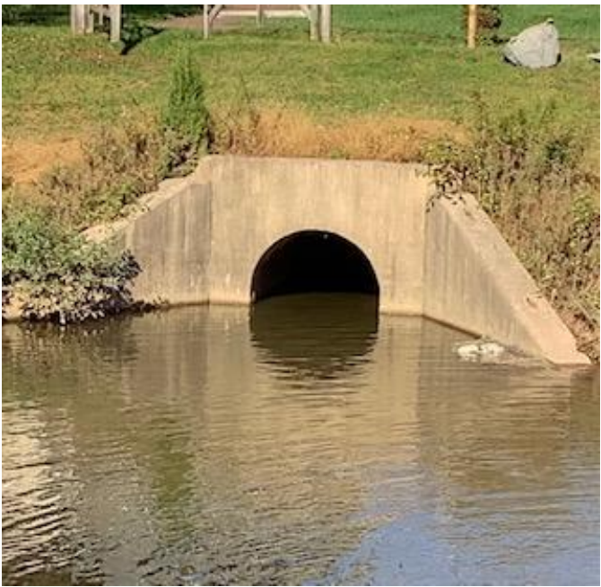
Pond 2 main inlet structure (one of two) is fed from Phase I and Phase 2 storm water systems.
